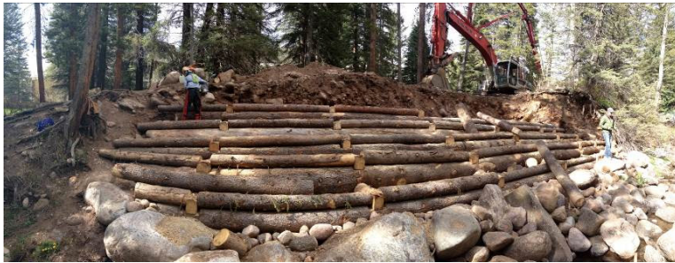
Bio-stabilization of a live crib bank with native riparian species designed by RiverRestoration was built to stabilize an actively eroding bank and provide safe access to a previously hazardous yet popular overlook of Gore Creek.
