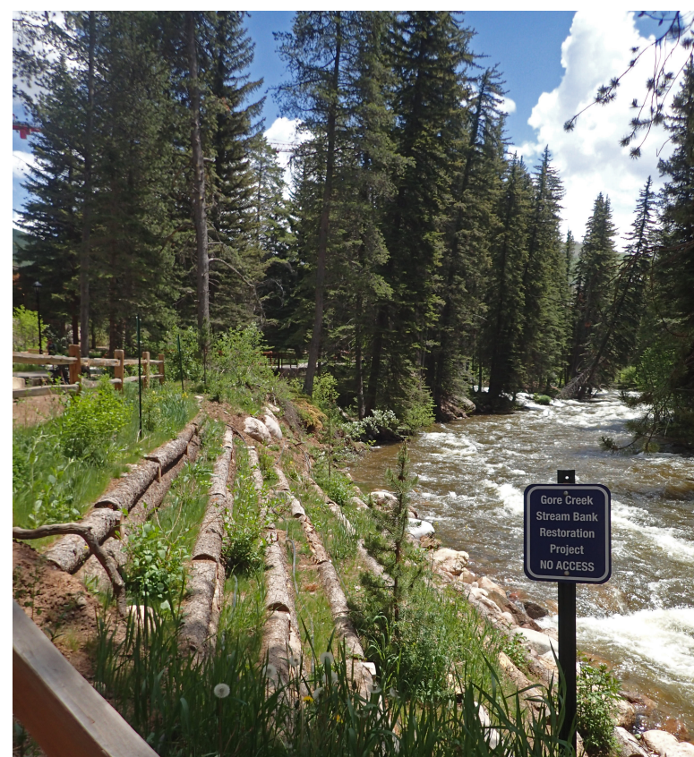
Bio-stabilization of a live crib bank with native riparian species designed by RiverRestoration was built to stabilize an actively eroding bank and provide safe access to a previously hazardous yet popular overlook of Gore Creek.
