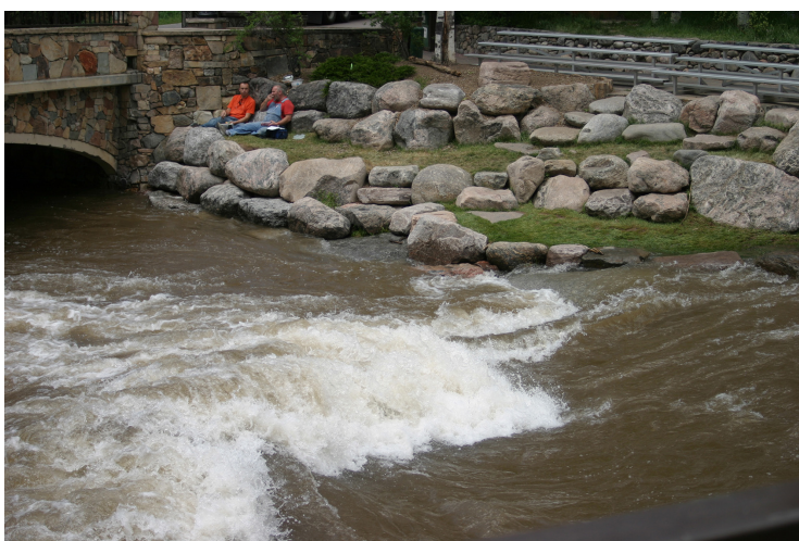
This photo was taken just after 100-year flood waters receded showing the RiverRestoration designed bank and whitewater feature in solid working condition
