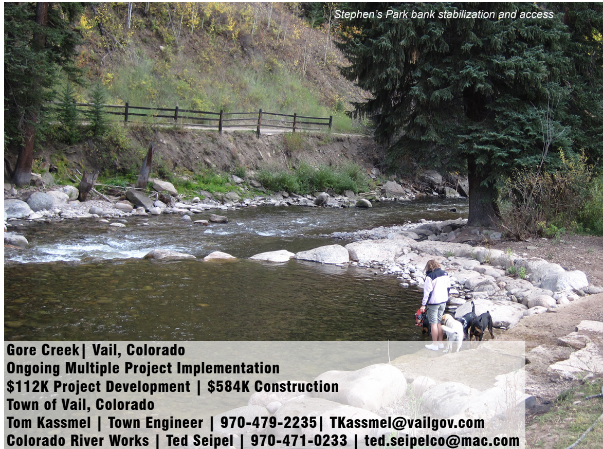
Bio-stabilization of a live crib bank with native riparian species designed by RiverRestoration was built to stabilize an actively eroding bank and provide safe access to a previously hazardous yet popular overlook of Gore Creek.
