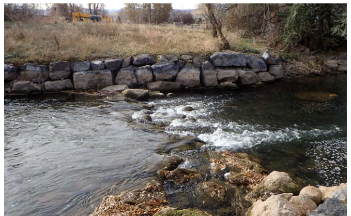
Close up view of the bottom rock-ramp structure at Pentz-Smith
