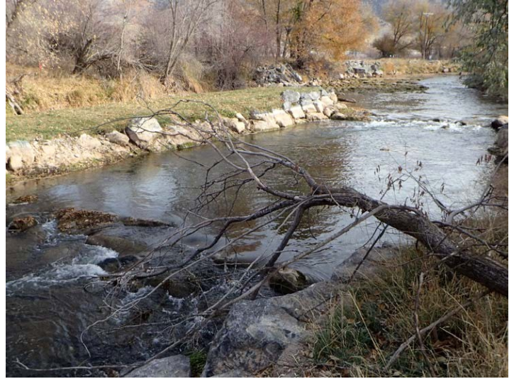
Pentz-Smith fish passage improvements after restoration include two grade control structures to reduce vertical drop over diversion structure and maintain upstream pool elevations
